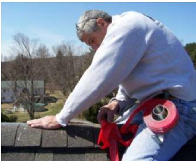
Applying ShockTape should be a “hands on” process. You will get a sense of how well the ShockTape is bonding or sticking to the surface. If it is not bonding well, stop the installation and correct the problem before continuing the installation.
