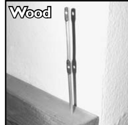
Double check installed post heights for masonry and wood installations.
