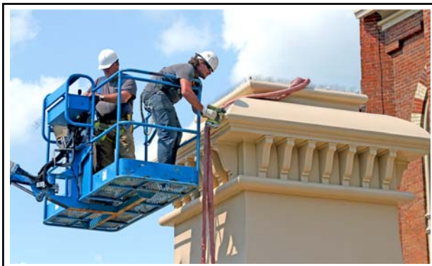
All of the Premium Nixalite Spike were fastened to the tower with the Bird Spike Mounting Hardware that was supplied with the Premium Spikes.
