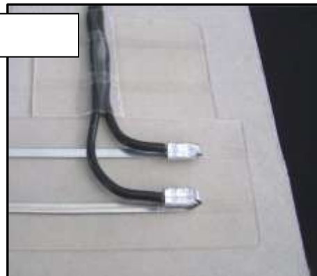
End Tap with wires dressed to the inside, secured by scrap tape.
