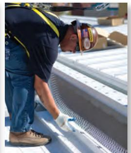
Premium Nixalite is the original and most successful bird barrier needle strip ever made. Made entirely of high grade stainless steel wire and strip, these barriers protect all types of surfaces from all pest birds and climbing animals. Premium Nixalite's applications are limited only by the imagination.
