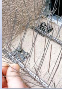
Glue Clip Installation
